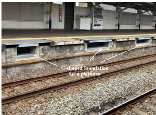
※ The photo shows a state before the installation of platform doors
